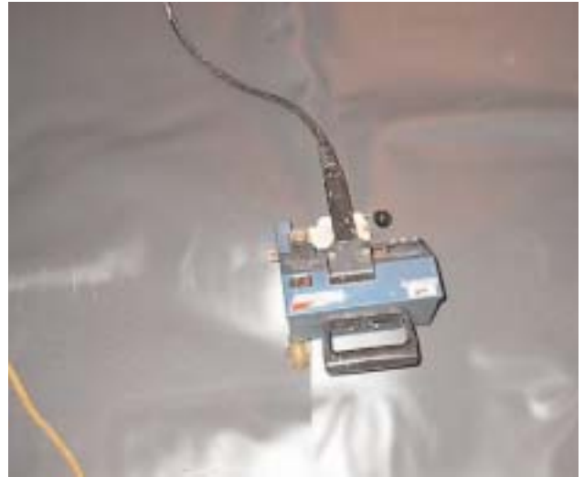
Photo 1b. Hot-wedge welding.
