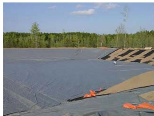
Details, testing and repairs were completed the following day. The 121,000 Sq. Ft. of 30 mil liner for cell two will be installed in June.
