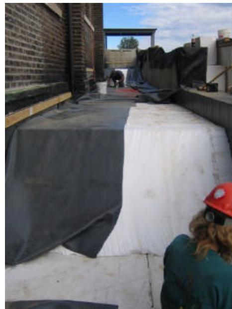
PVC was used in a 10' wide, 20' deep and 92' long (3M x 6M x 28M) cavity filled with Geofoam.
