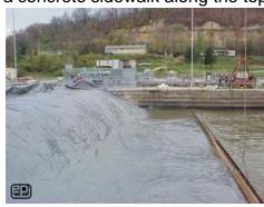
of the dam. The panel was then positioned by lowering the beam along the face of the dam underwater until the full width of the panel was unfolded in place. Each end of the liner was then attached with batten to the walls
