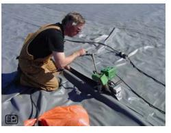
one on May 24, 2002. The panels were installed and thermally welded by one crew, with one welder, in one day.
